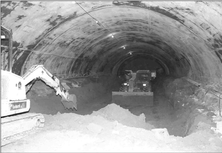
Figure 3. “Belgian” tunneling method, Line H, 2000.
