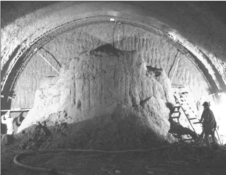
Figure 4. Full face excavation, Line B, 2004.
