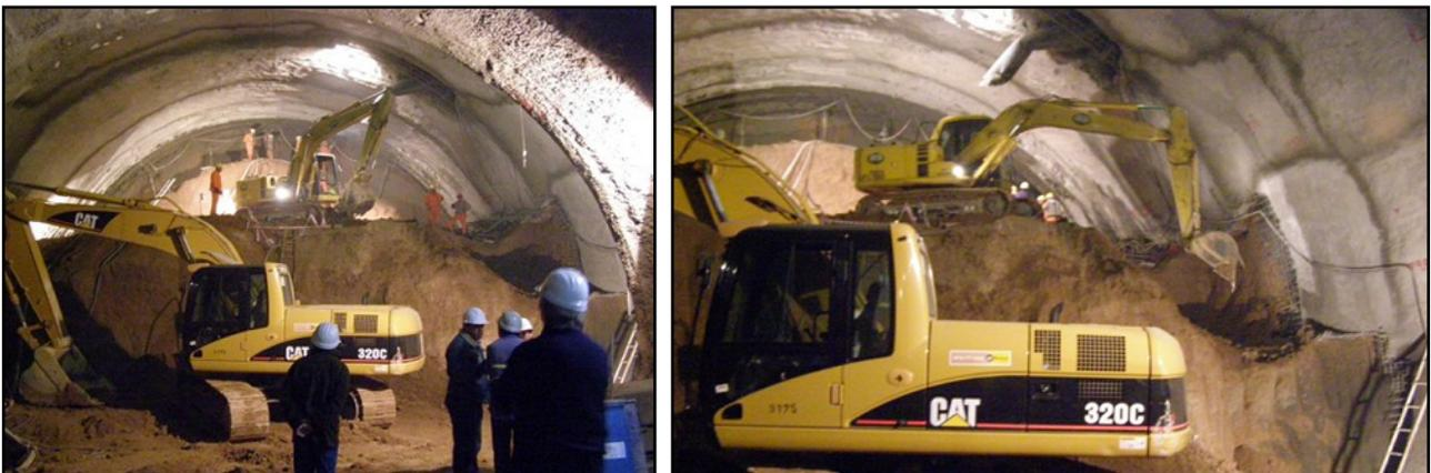
Figure 14. Excavation of bench #2, Corrientes Station. Notice the position of the upper backhoe excavator.
