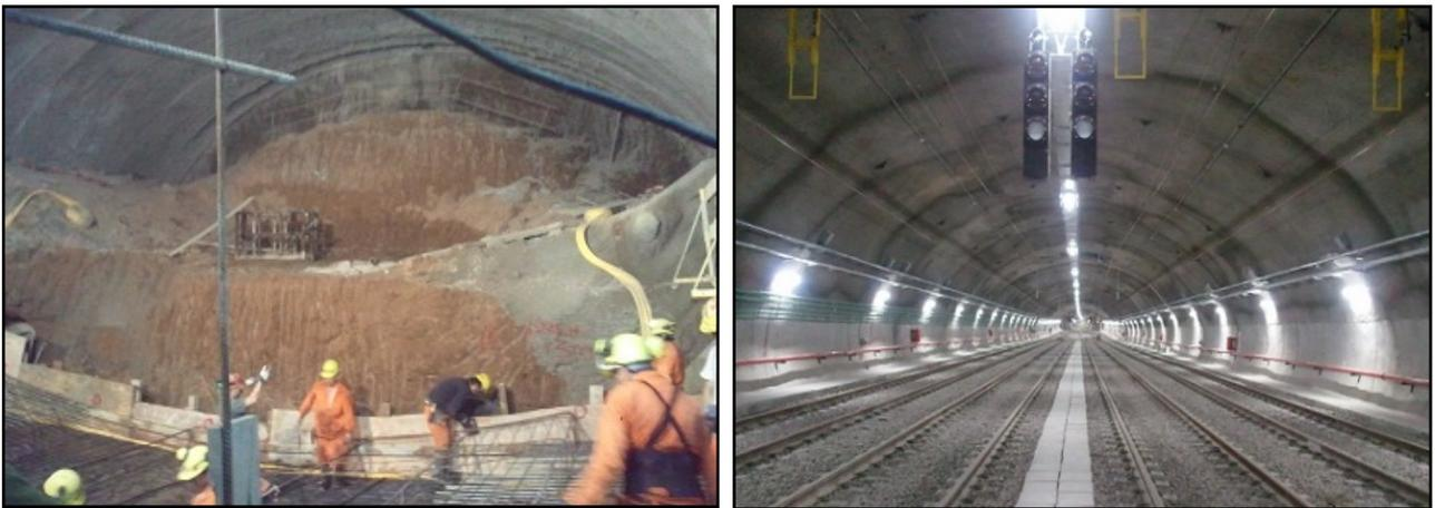
Figure 19. Warehouse cavern, Line A. Construction of invert and final view.
