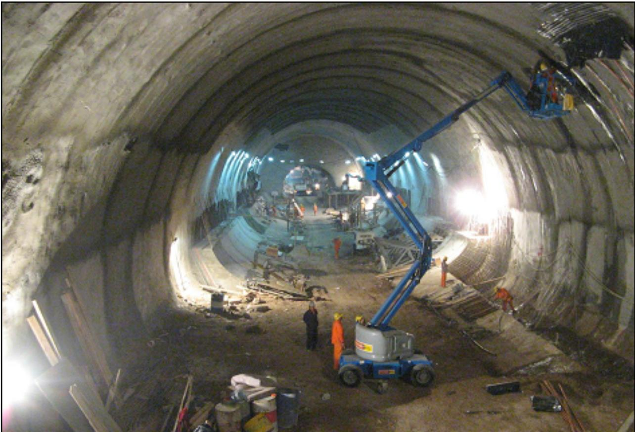
Figure 15. Corrientes Station. Construction of secondary lining as seen from the upper bench (position of the camera).
