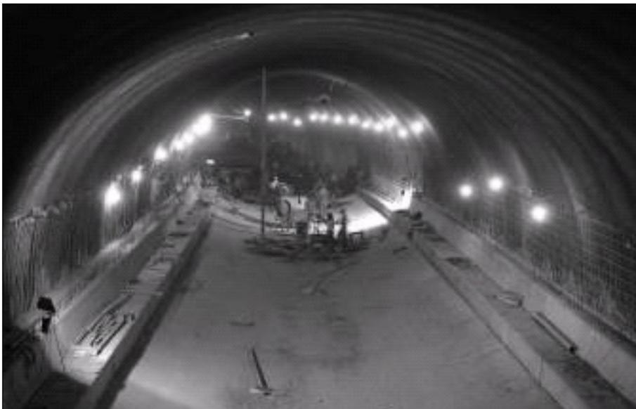
Figure 6. Tunnel after placement of the invert, Line B.
