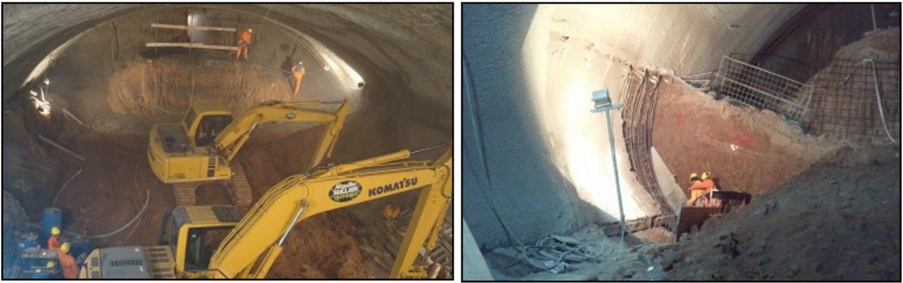
Figure 18. Warehouse cavern, Line A. Face and bench excavations.
